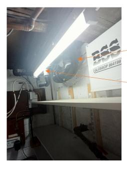
Waste pipes from ground floor WC – need boxing in and insulating.
