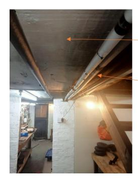
Lath and plaster ceiling to be removed, insulated, and reboarded.
