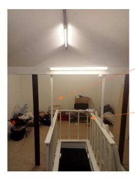
Loft floor to be lifted, 400mm of insulation added and floor relayed on legs.
