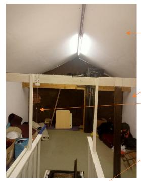
Stud walls and ceilings to be removed, insulated between and over rafters with 100mm wood fibre insulation, reboarded and plastered.
