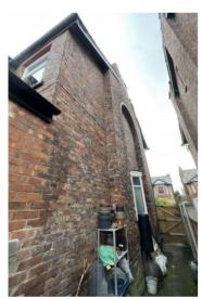
achieve greater energy savings, as well as keeping the floor joists and thermal mass of the masonry inside the heated envelope. To maintain the character of the building the external chimney stacks could remain exposed, insulating them with glass beads inside the chimney, and then EWI installed to the surrounding wall areas.
